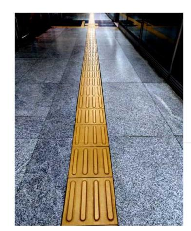
Tactile Paving is a system of texturing the floor ground surface to assist pedestrians who are visually impaired complete their journey with ease and confidence. This is achieved by installing a specialized product called PU Tactile. These tiles provide guidance and help convey important information such as clues, directions or warnings.
